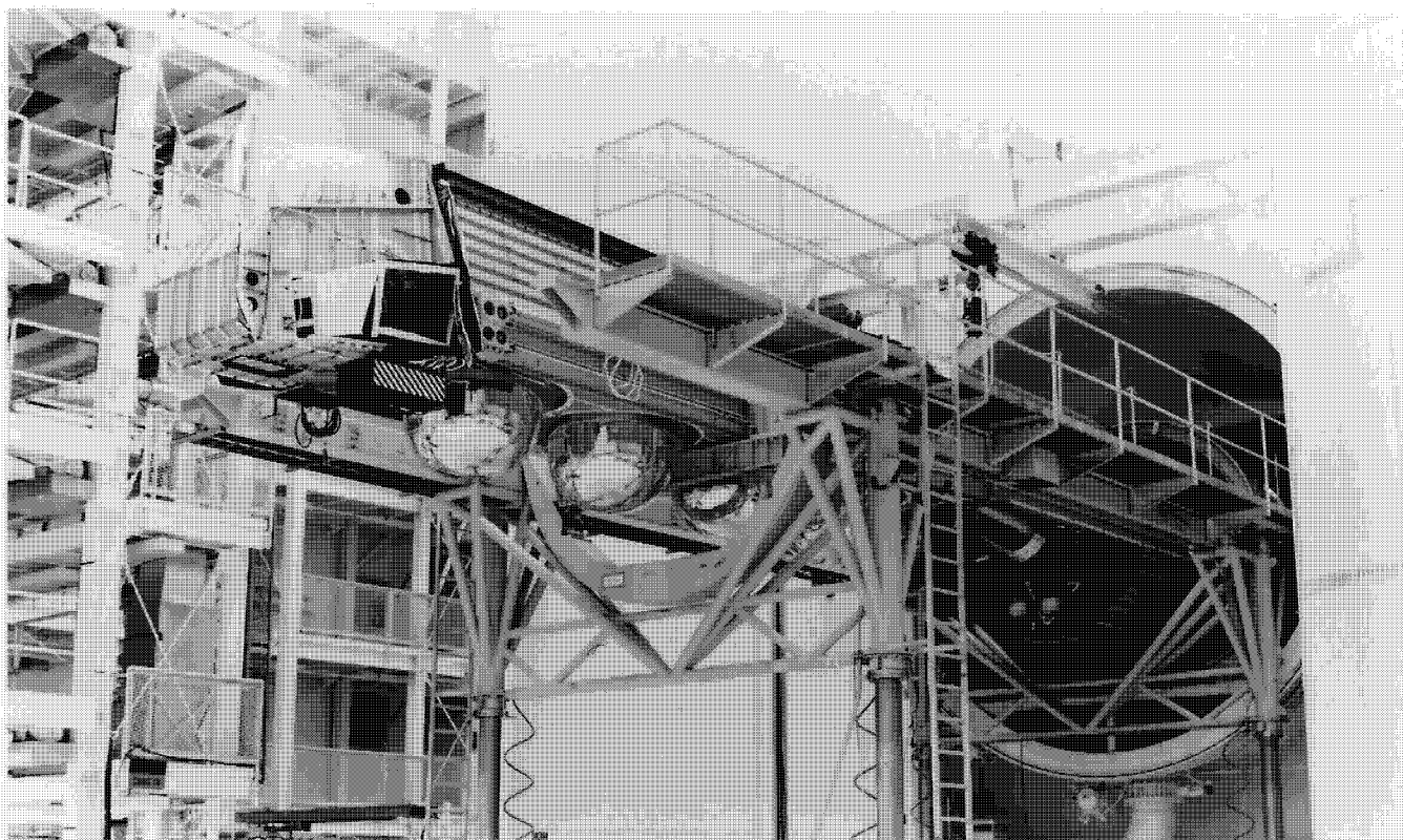
Fig. 2-28 — SV entering vacuum chamber
