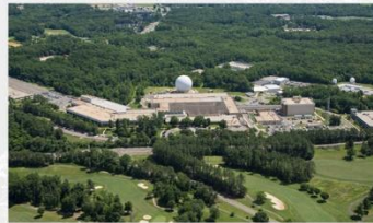
Aerospace Data Facility – East Fort Belvoir, Virginia
