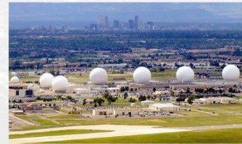
Aerospace Data Facility – Colorado Aurora, Colorado
