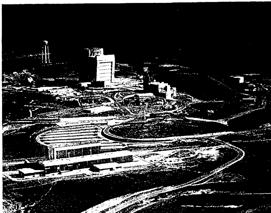
EXISTING SLC-6 FACILITIES AND ADJACENT HILLS VIEWED FROM THE NORTH-NORTHWEST
