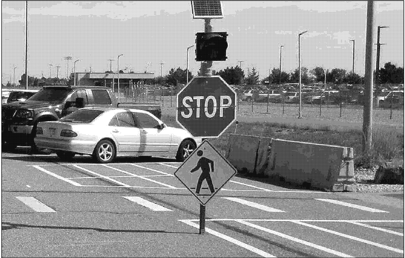
(U) Figure 4-3: Example of Flashing Beacons and Multiple Messages on a Shared Post
