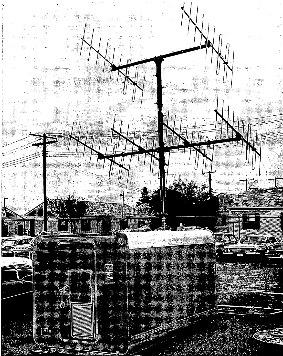
Fig. 1 - Primary Hut showing YAGI Antenna System installed
