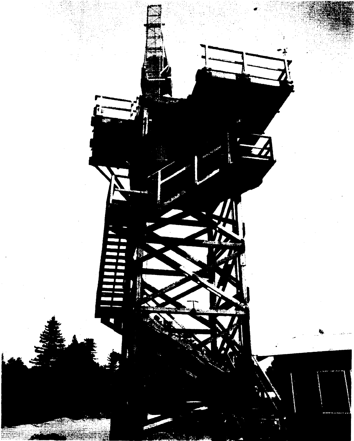
Figure 2.1.5.2 - Radar Antenna on Bore-sight Tower
