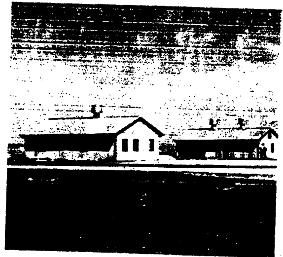
Figure 3. Construction progress at the Southeast Africa tracking station (Atlantic Missile Range Station 13) near Pretoria. The tracking station support buildings and the power vans (left) and the communication building (left) and power supply building (right) (above) are nearing completion. This station will be ready to record AGENA second-burn data on the MIDAS III flight.
