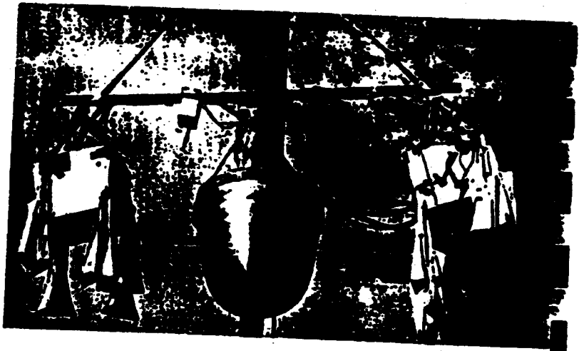
Figure 3. Test capsule (left) suspended from the balloon that will carry it to 100,000 feet altitude. Closeup (above) of test capsule and telemetry equipment which provides flight data and through which the release command is received. The ablative shield which protects the capsule from the heat generated during high speed re-entry into the atmosphere is shown. The external surface of the shield peels off under the intense heat of friction, thus dissipating the heat and protecting the capsule. The capsule and parachute are contained within this shield. Aerial view (right) of the capsule during descent over New Mexico. The parachute deployed at approximately 55,000 feet altitude. Capsule immediately after impact (lower right). Closeup of the capsule and parachute (lower left). An impact at sea would cause little damage to the capsule structure.
