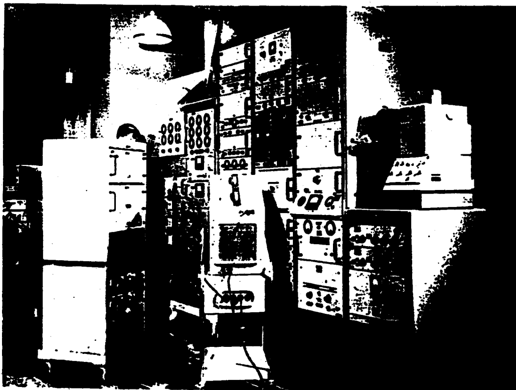
Figure 9. The first set of E-1/E-2 ground reconstruction electronics (GRE) equipment installed in the Vandenberg Air Force Base missile assembly building.
