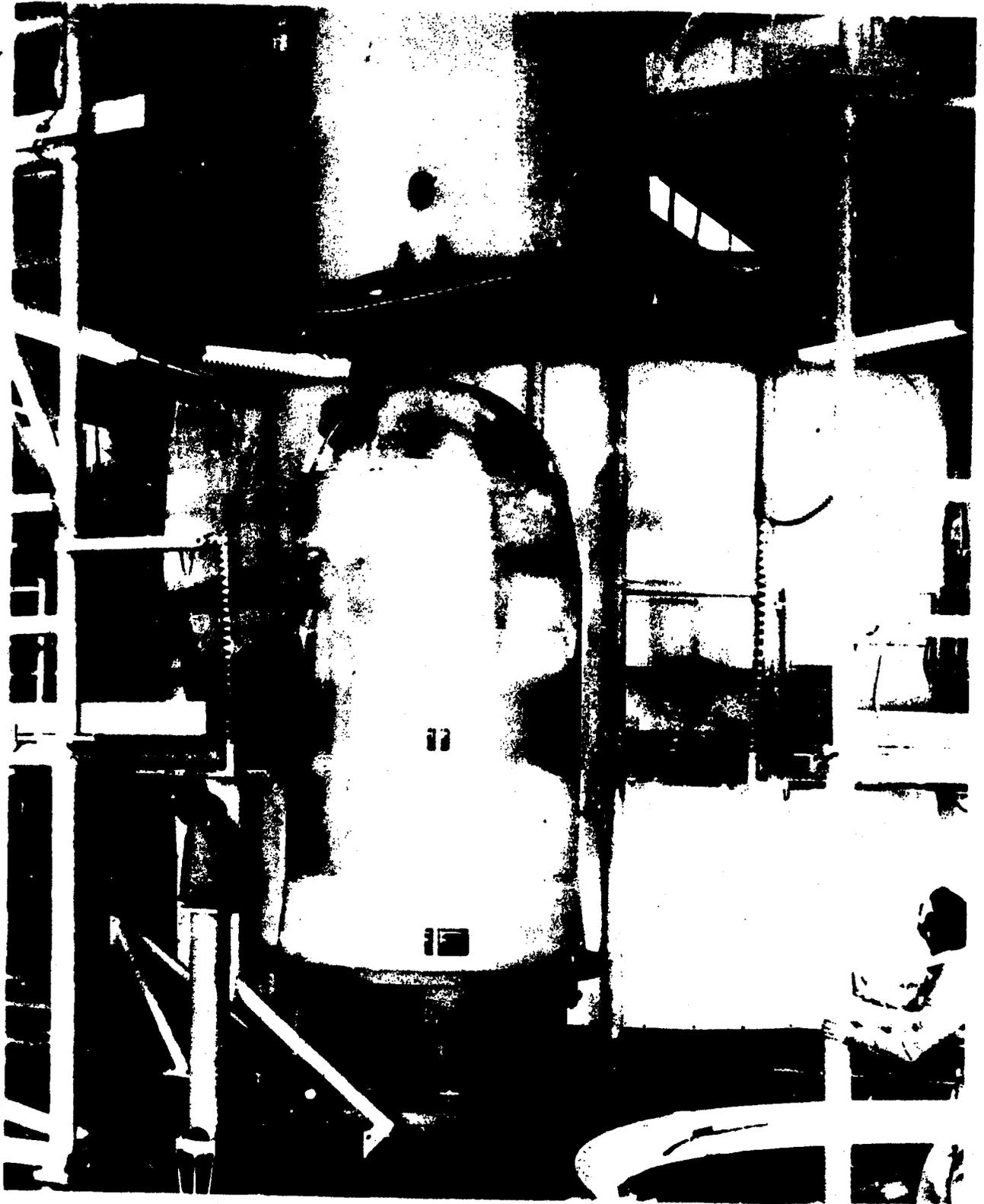
Figure 3. Stacking of forward mid-body sections, prior to mating with the aft-body section. (WDPC-58-24)
