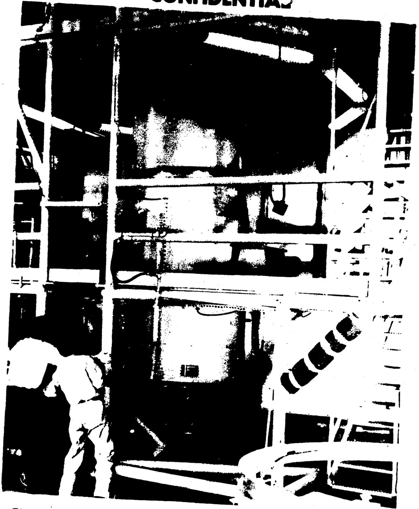
Figure 4. Mating of the forward mid-body sections with the aft-body section.
